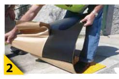
While standing on the mat to prevent movement, remove one section of the paper backing.
