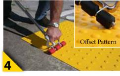
To insure a secure bond is achieved, roll the mat both lengthwise, widthwise and most importantly along the edges, with the handheld RediMat™ Roller. For mats with an offset pattern hold the roller at a 45° angle and use the outer roller pad to roll between the domes diagonally from front to rear and along the edges.
