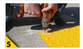
Using the drill and a 5/32 in. masonry bit, drill through the pre-drilled holes into the concrete to a depth of 1 1/4 in. If the mats are trimmed so a pre-drilled hole is removed, a new hole must be drilled in the mat using a 3/8 in. standard drill bit, 2 in. from the side edge and 1 in. from the beveled edge.
